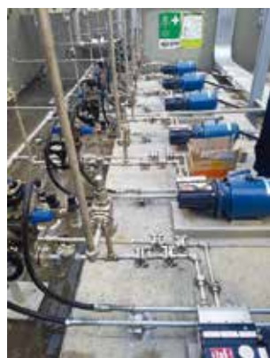
Aqueous ammonia supply pump
