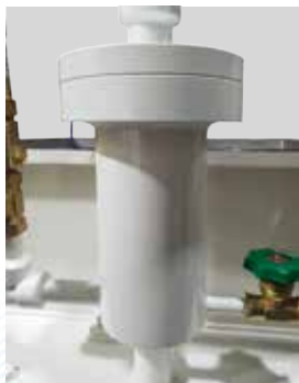
Differential pressure type (Liquid gas overflow prevention device)
