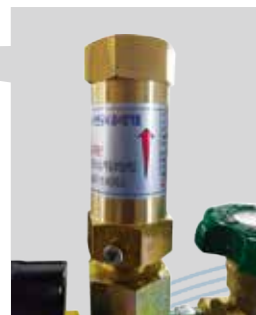
Safety valve (Discharge device of abnormal pressure)
