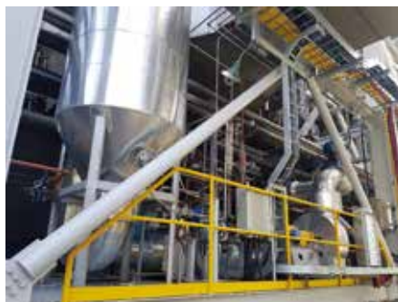
Aqueous ammonia E-Vaporizer
